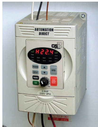
Photo 7—In the 20th century, motors were either “on” or “off”. It's a new world now with the Variable Frequency Drive (VFD).
